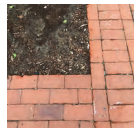
This flat edge around a tree pit allows rainwater to reach tree roots.
